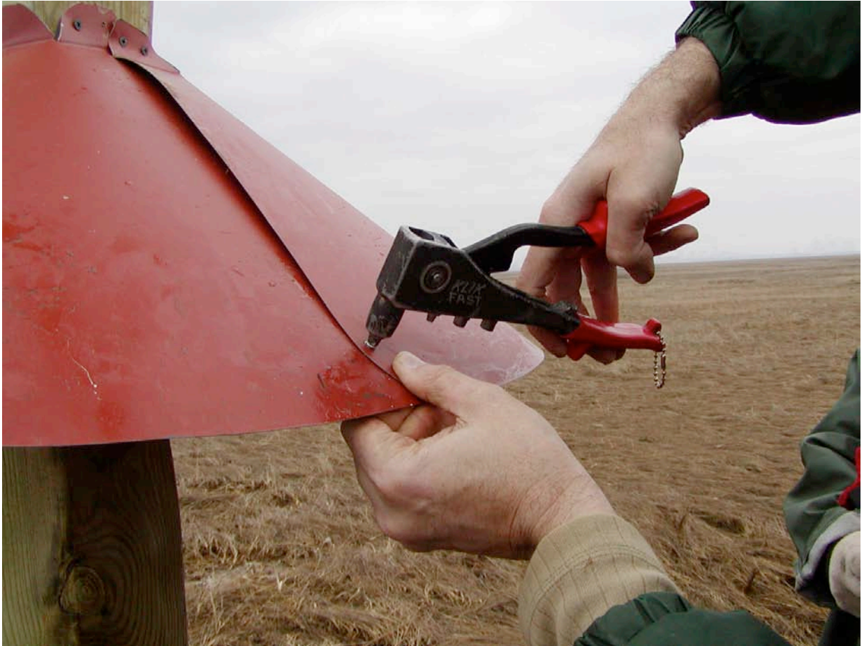
Inserting pop rivets in holes
