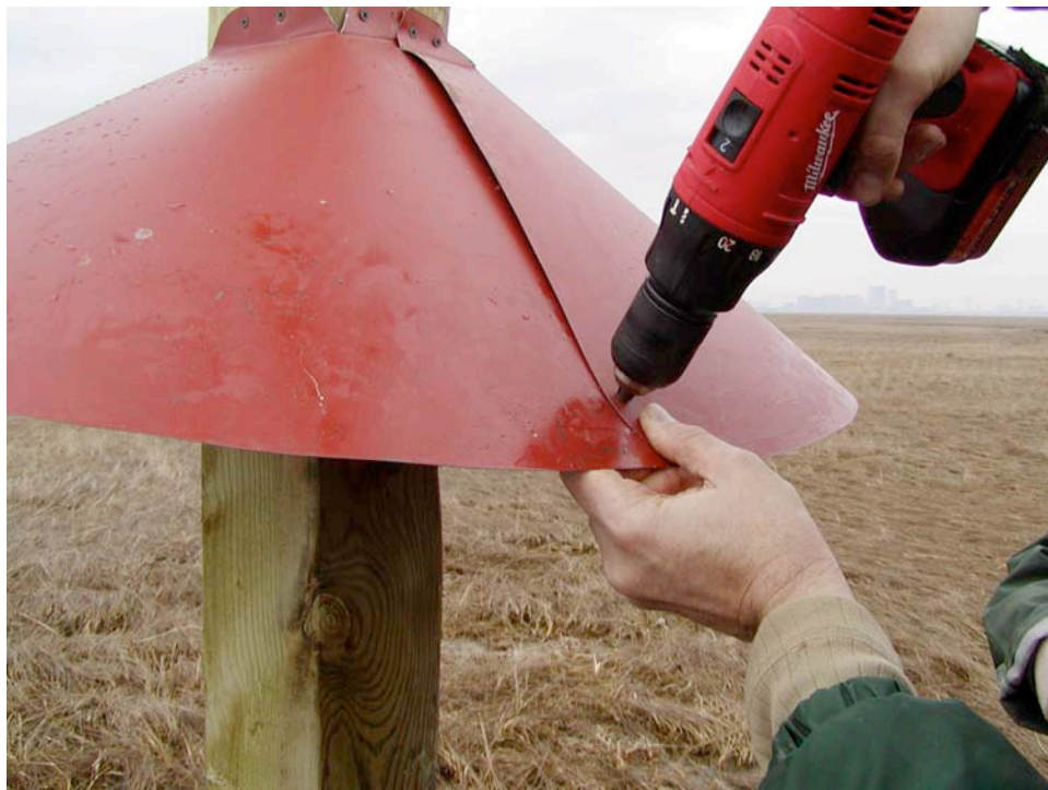
Drilling holes for pop rivets along open seam
