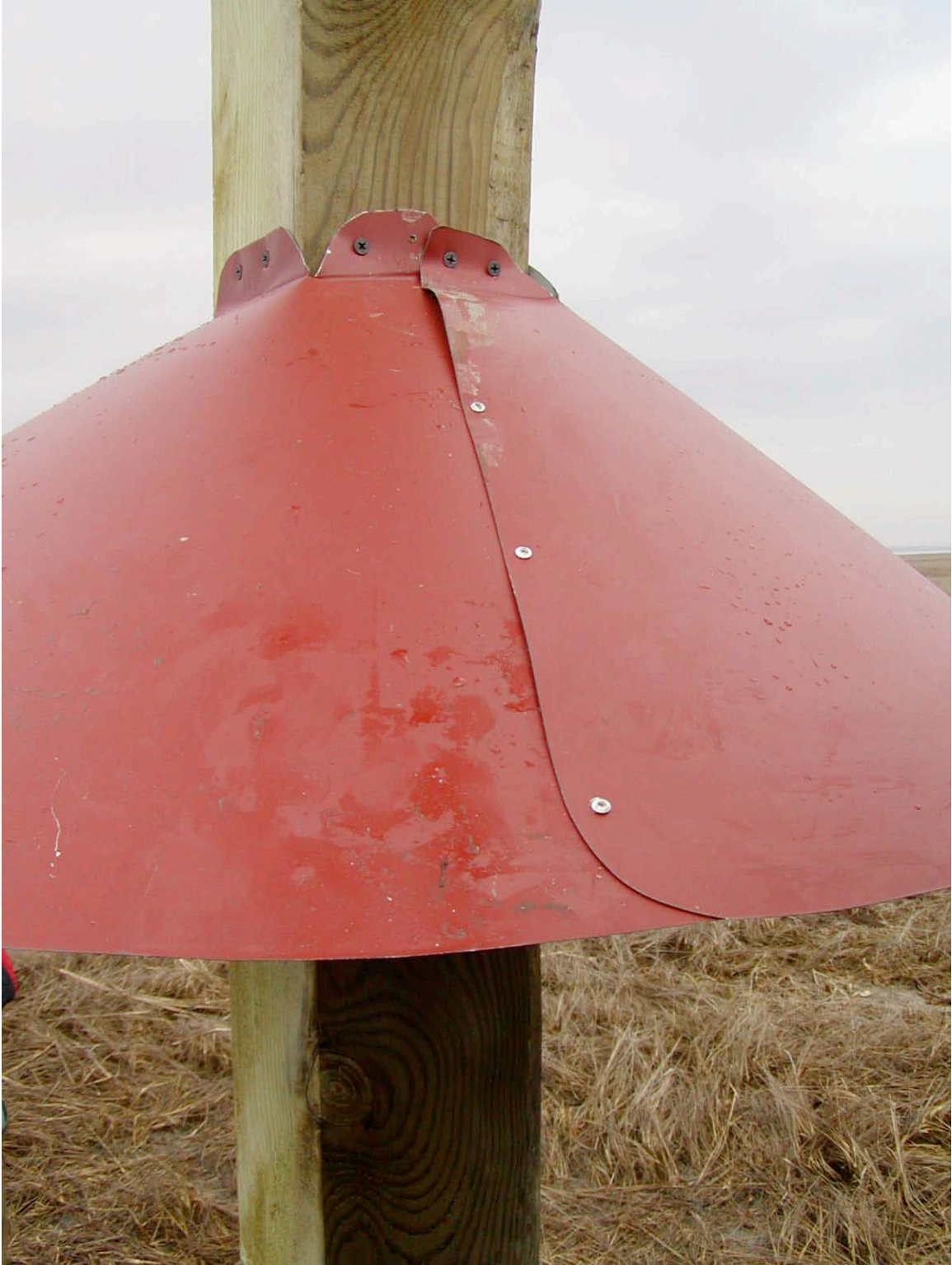
Rivets in place
