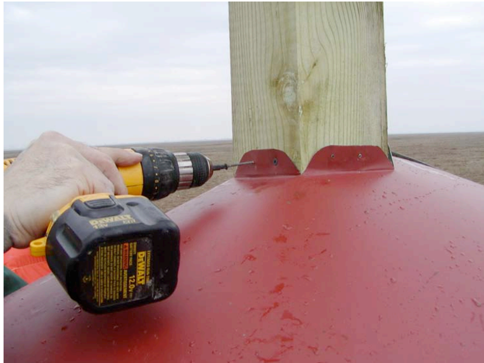
Screwing the guard at two spots on each side of the nest
