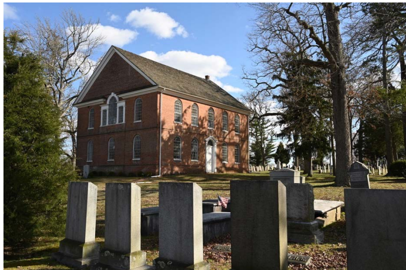
Bridgeton's Presbyterian Meeting House, built in 1792, is known as the Historic Broad Street Church.
