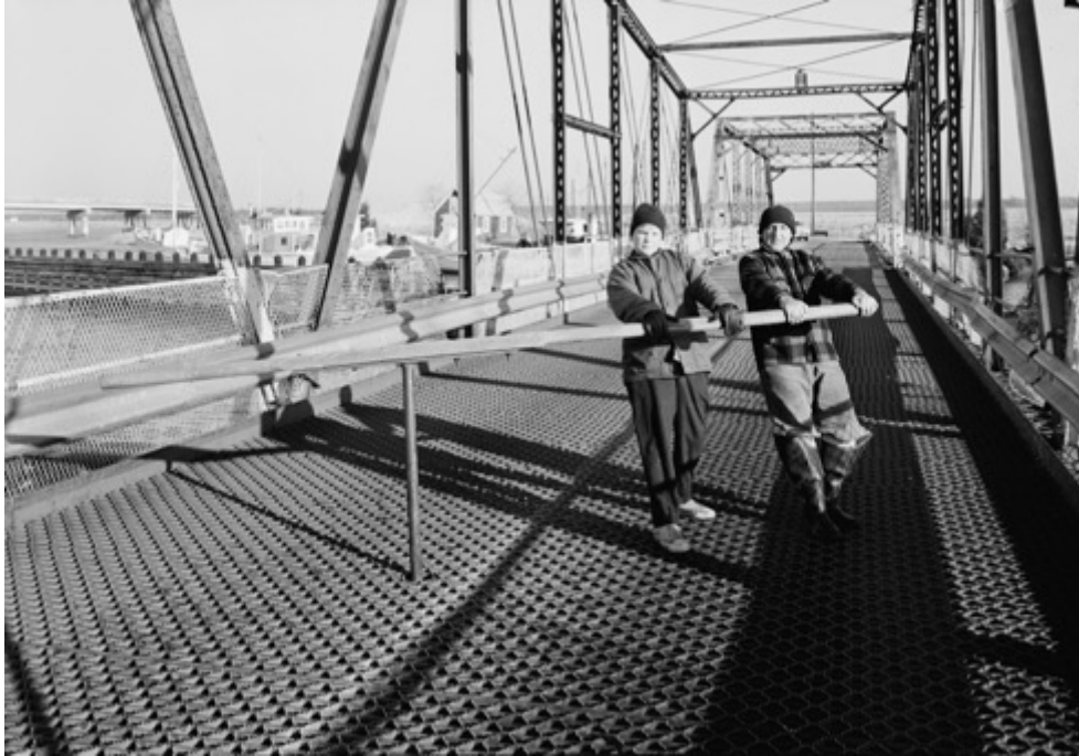
Albert Reeves (right), the last bridge tender, and Wally Hales open the Pratt Through Truss Swing bridge that once crossed the Maurice River. This bridge's key is on display at the Mauricetown Historic Society's headquarters in Mauricetown. Note the present-day Causeway Bridge in the background. Photo: Library of Congress, Dean and Westbrook.
