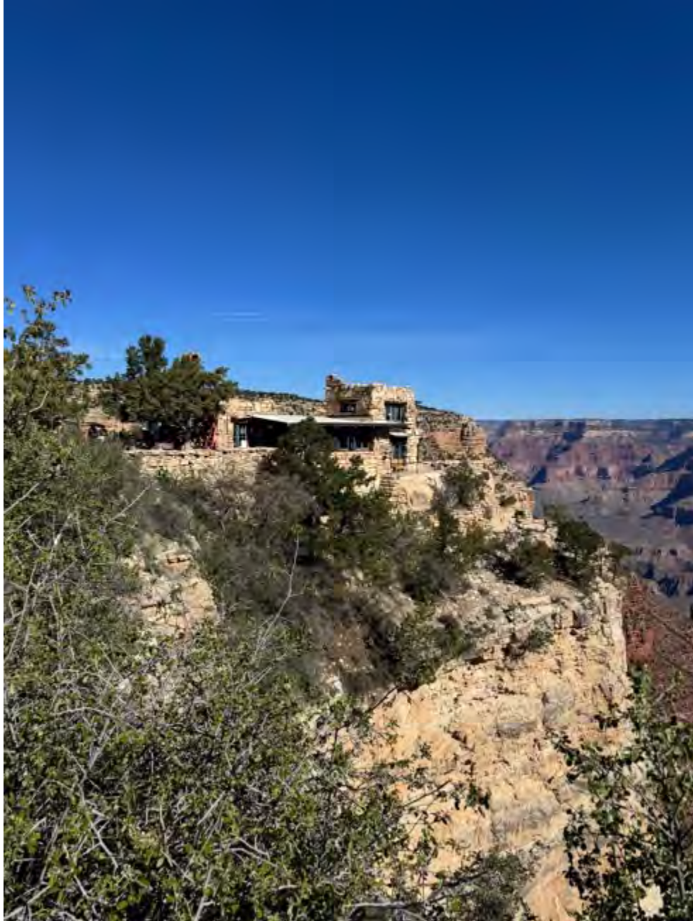
Architect Mary Elizabeth Jane Colter's Lookout Studio (1914) designed this building for Fred Harvey. Colter's pioneering and distinctive style helped to shape the architecture of the Southwest and its national parks. The locally quarried limestone makes it appear like part of the canyon wall. Photo: JMG
