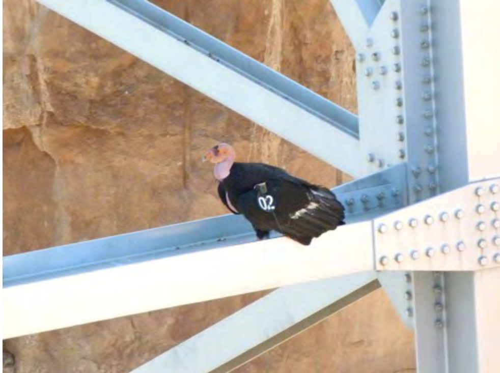
Historic Navajo Bridge is the site of a California condor roost. Photos by Heather, Trip Advisor.
